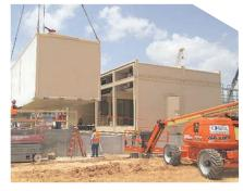
Modular buildings from 50 sq. ft. to 15,000 sq. ft. can be manufactured off-site, transported to the project location and assembled. This provides all the amenities of traditional construction with the benefits of modular.
